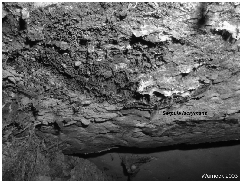
Figure 2: Serpula lacrymans fruiting body on a stone slab in the crawlspace of a century old building in Southern Ontario
